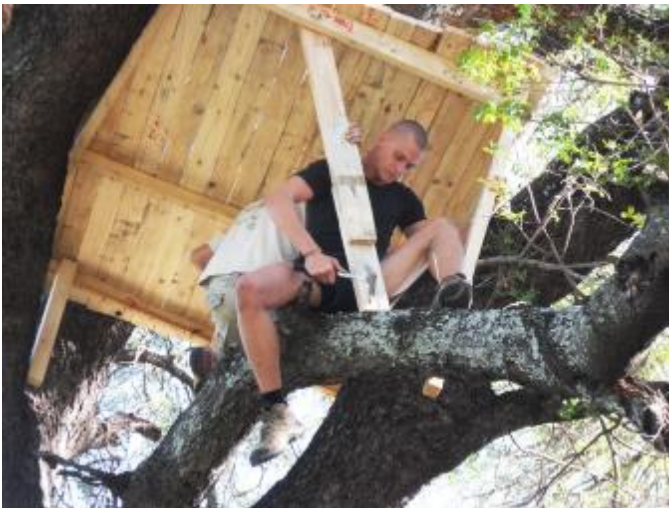
Bart and Jamie hard at work securing the deck
