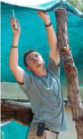
Stitching netting for the carport
