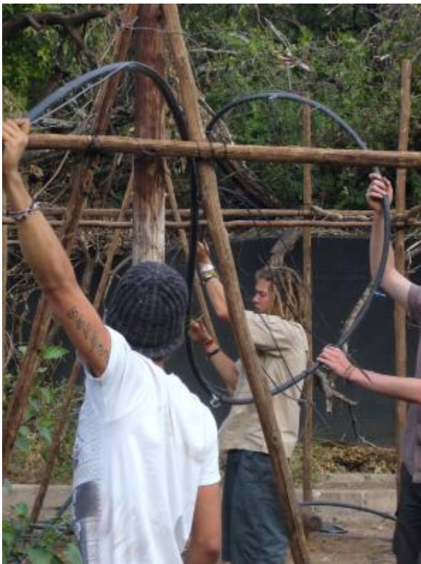
The volunteers repairing the existing structure
