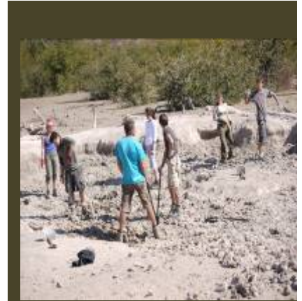
Digging a new elephant watering hole.
