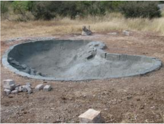
Nearly ready for water
